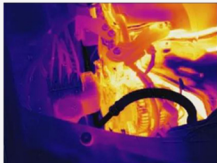
Mechanical equipment inspection
